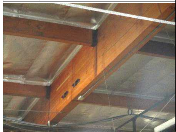
6. Wood purlins and glue-laminated girder.
