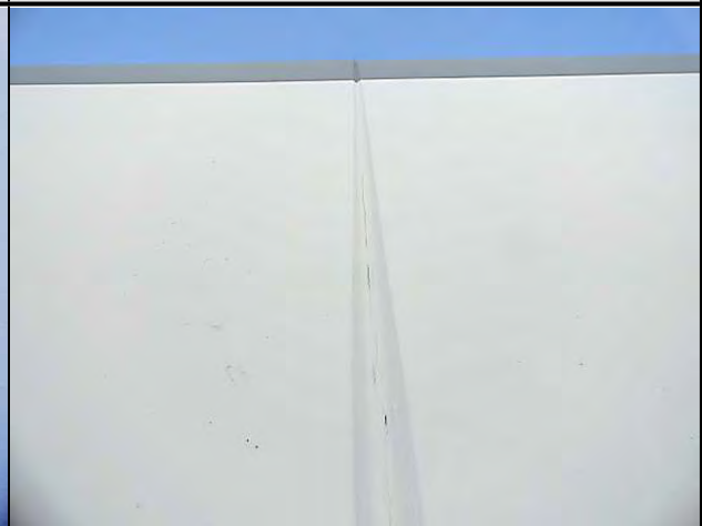
Typical condition of vertical panel joints
