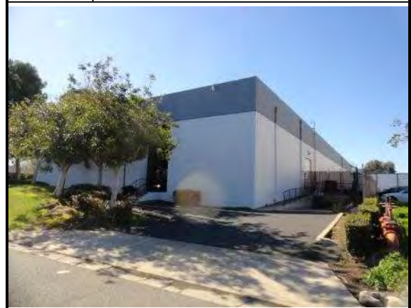
5. Northeast corner elevation showing east side and north rear facades
