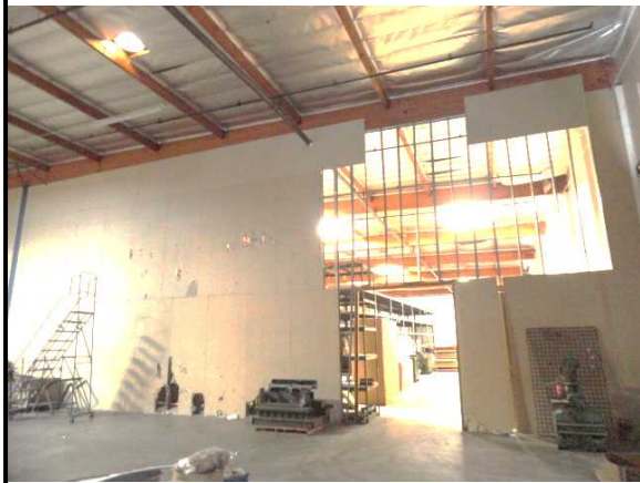
38. Occupancy separation wall between main tenant space and sub-tenant space
