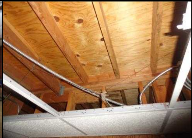
Office area second floor deck framing
