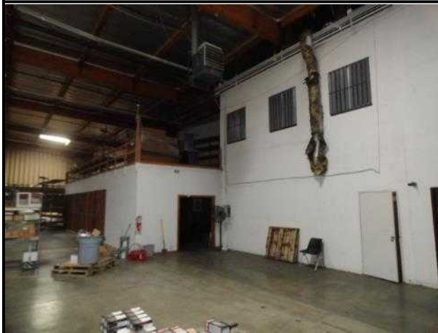
Office area separation walls seen from the warehouse area
