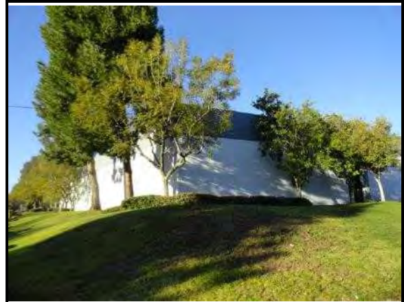
4. Southeast corner elevation showing front south and east facades
