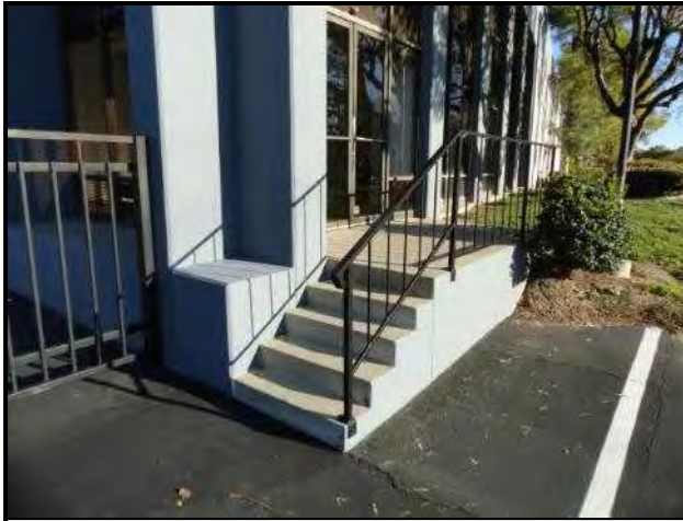
Concrete stairs and steel railings at southwest entrance
