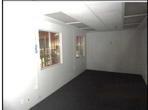
48. Typical second floor office area finishes
