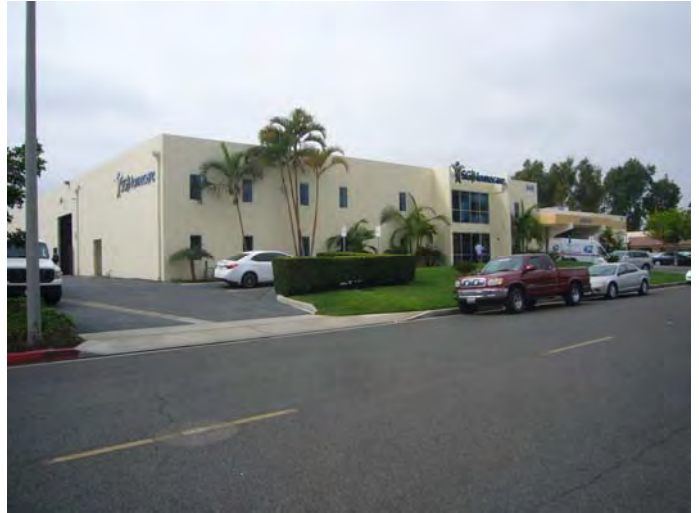
2) View of the adjacent property to the northwest.
