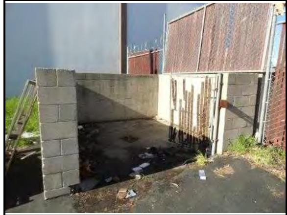
22. Trash bin enclosure at northwest corner of site
