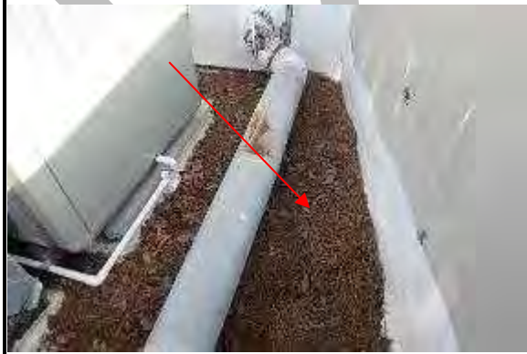
3. Pine needle debris on membrane
