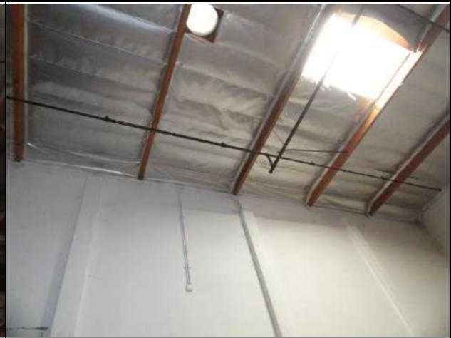
Roof deck framing at the exterior wall panels
