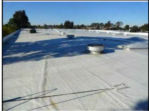
28. Overview of roof
