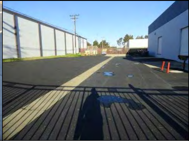
Storm water drainage swales
