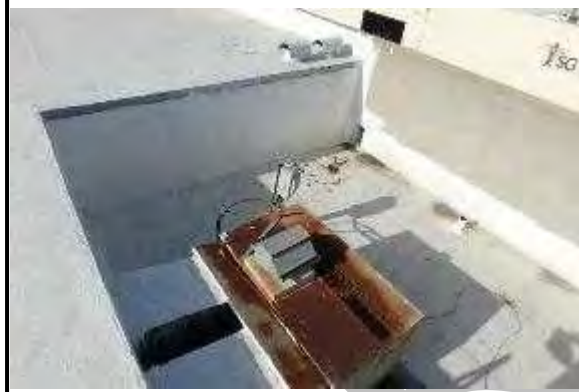
2. Overview of Roof Section 02
