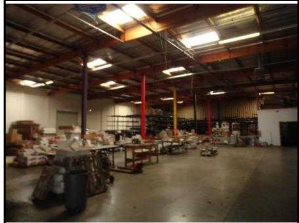
35. Typical roof framing in the warehouse area
