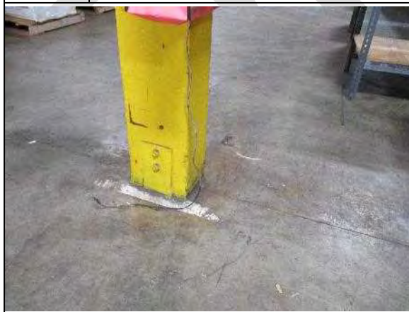
9. Base of interior wood column to concrete floor slab.
