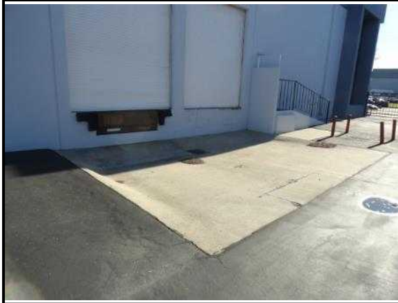
19. Typical apron at loading docks
