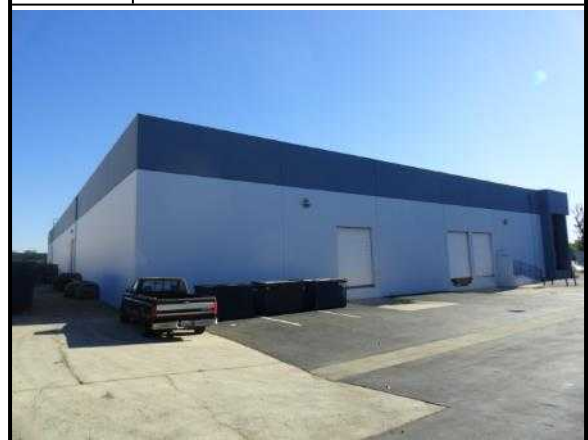
6. Northwest corner elevation showing west side façade and north rear facade
