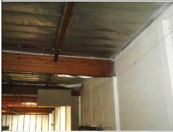
8. Glue-laminated girder on concrete pilaster at exterior wall.
