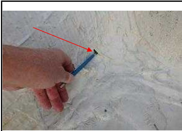
7. Open pin holes on return
