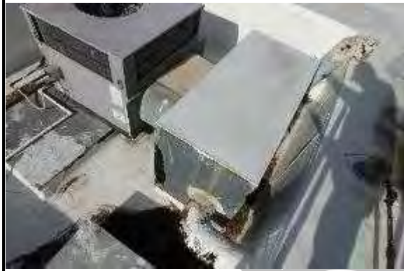
2. Overview of Roof Section 03
