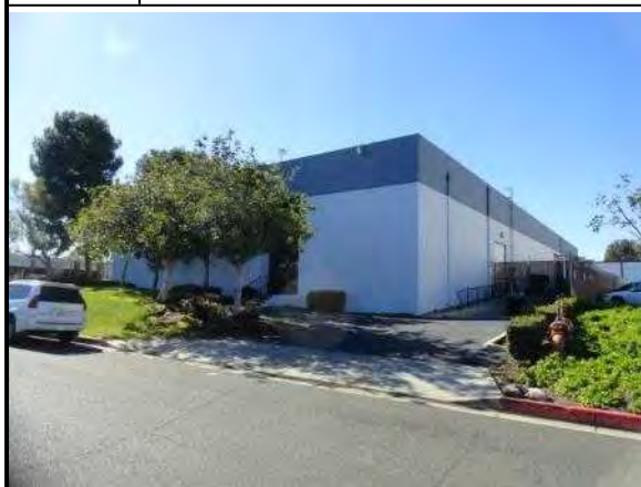
2. Northeast access drive and street view of the property
