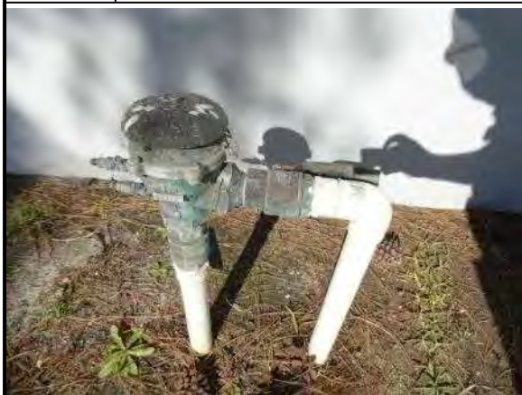
26. Landscape irrigation system backflow preventer
