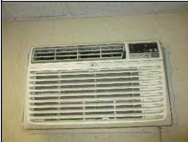
Figure 2.4.3 – Supplemental thru-wall AC
