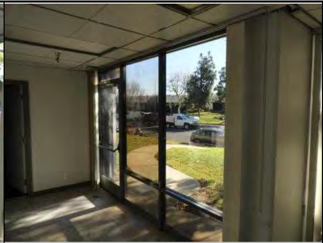
Ground floor office area secondary egress doorway
