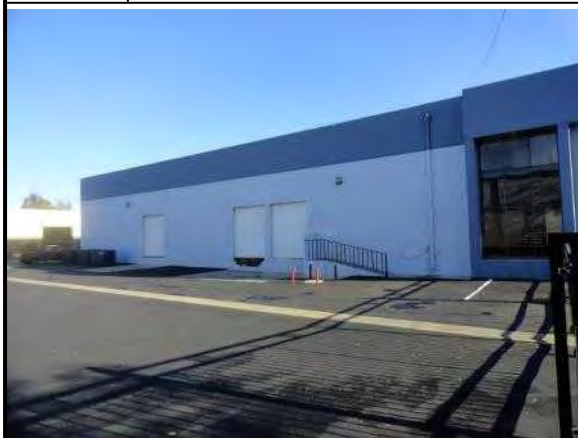
14. West façade showing three tailgate high loading docks
