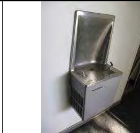
Figure 2.1.6 – Water bubbler
