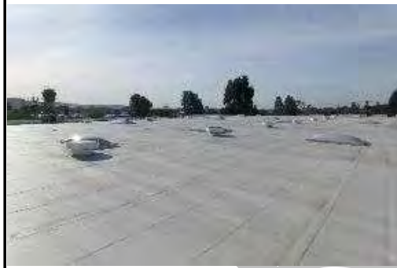
2. Overview of Roof Section 01
