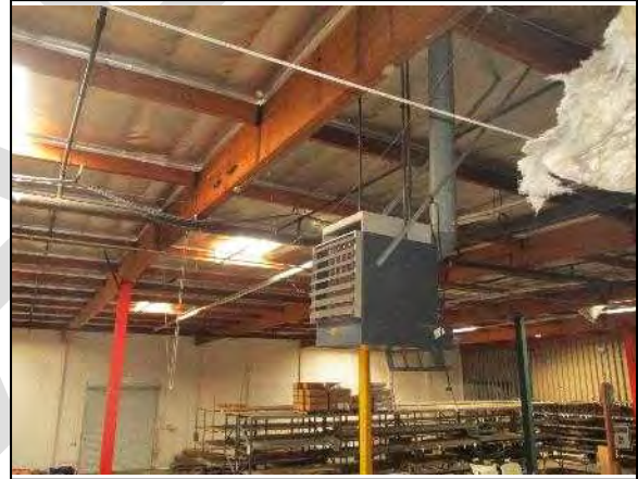
5. Underside of roof framing. Note diagonal bracing of HVAC unit.
