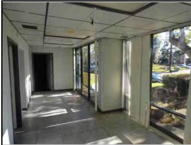
Typical office area finishes on ground floor
