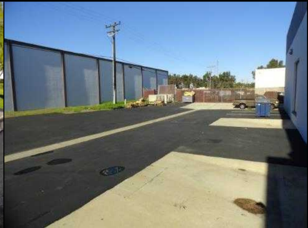
Power is provided from pole-mounted transformers with secondary feeders underground to the main switchboard in the warehouse area
