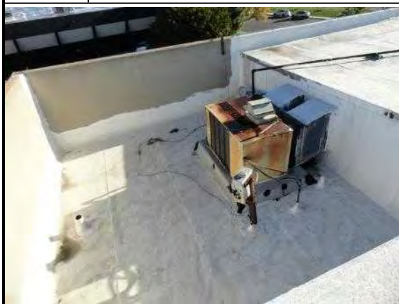
33. Roof in mechanical well over northeast office area
