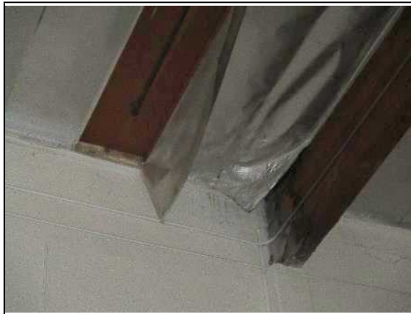
7. Glue-laminated girder on concrete pilaster at exterior wall.
