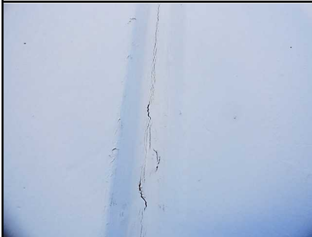
Typical condition of vertical panel joints
