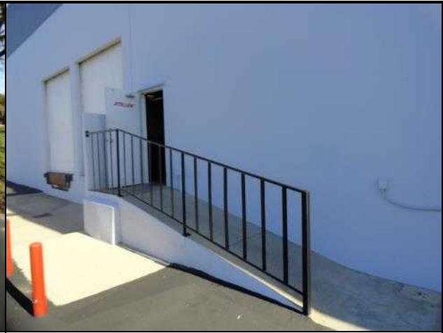
Concrete ramp and railing into warehouse area on the west elevation
