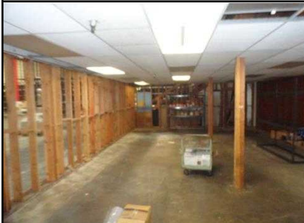
Office area framing
