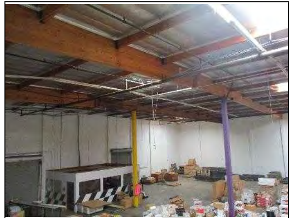
4. Interior of warehouse space.
