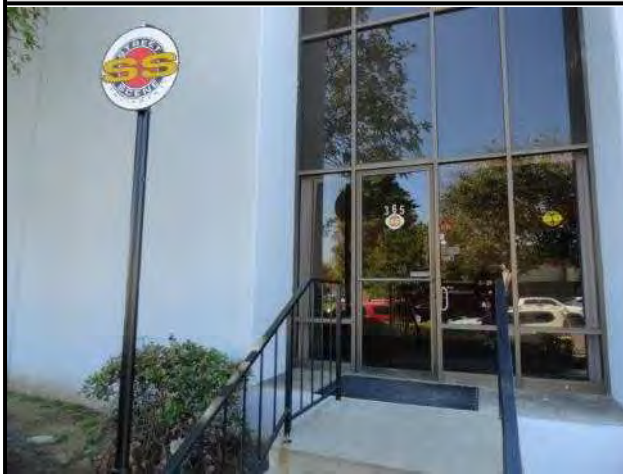
Concrete stairs, railing and signage at the northeast building entrance
