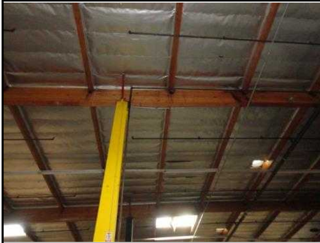
Detail of roof structure
