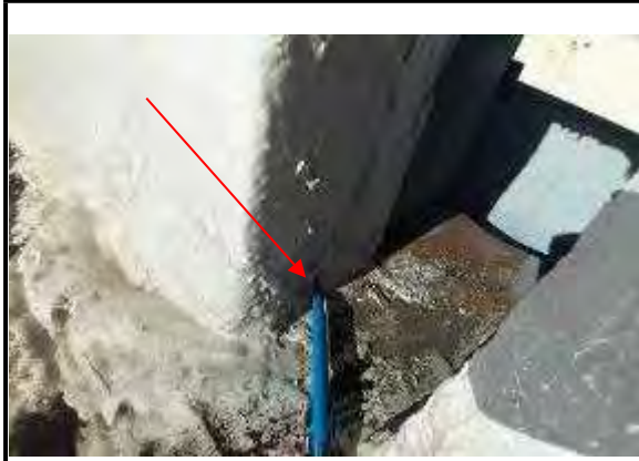
7. Voids in silicone coating
