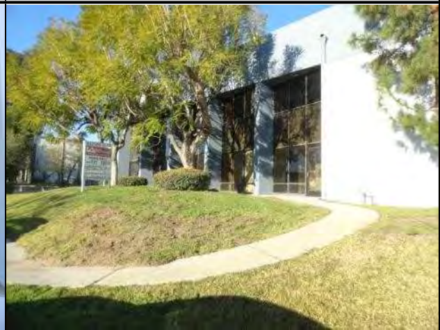
Concrete walkway leading to secondary entrance to the southwest office area
