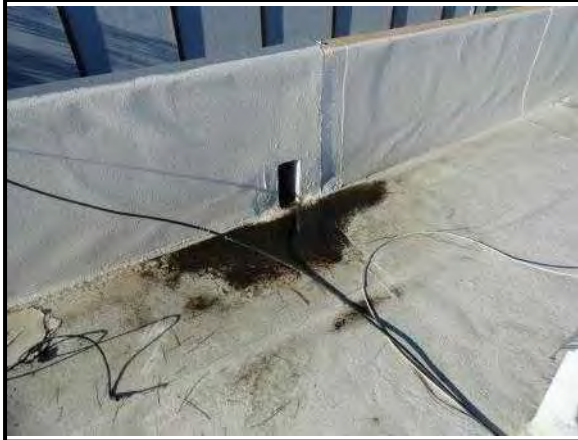
31. Typical parapet drain scupper
