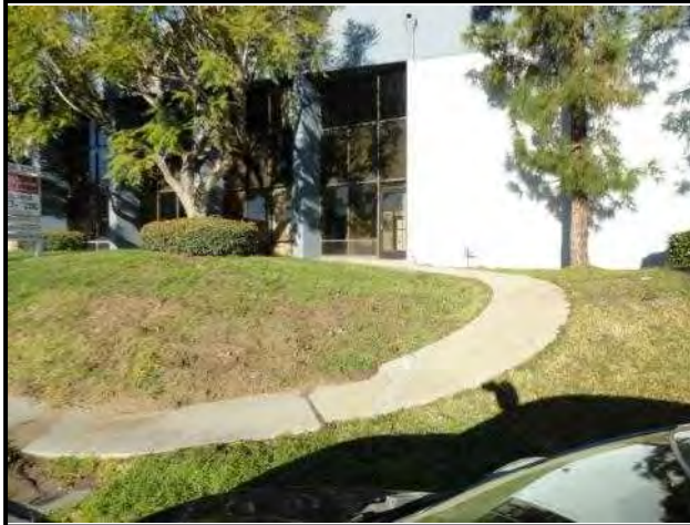
Secondary entrance and stairway egress at the southwest office area
