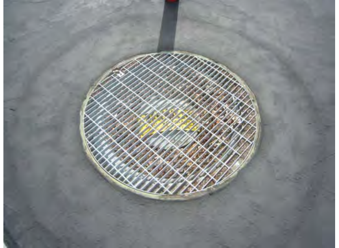
6) View of the electrical transformer vault.
