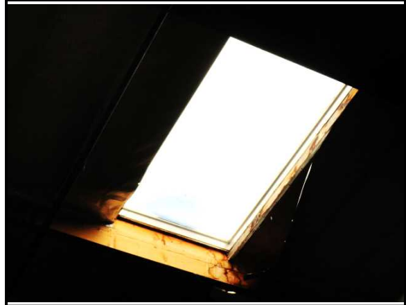
34. Typical roof skylight seen from inside the warehouse area showing no fall protection
