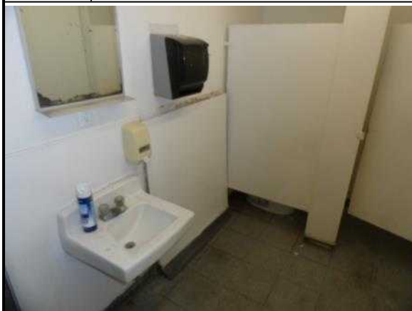
45. Typical restroom finishes and fixtures
