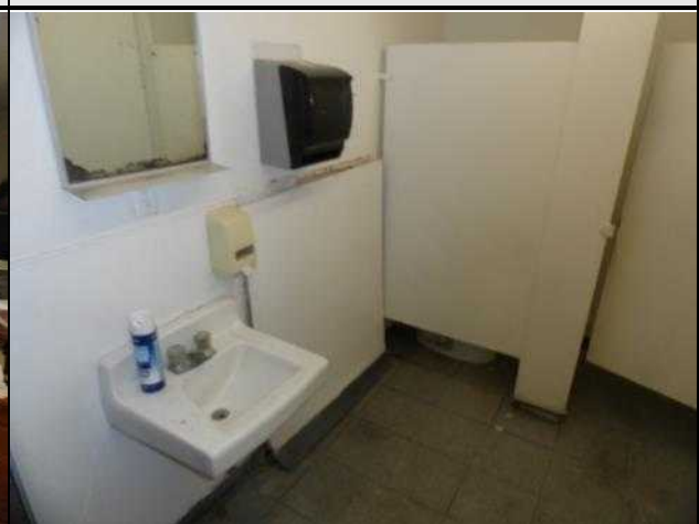
Typical restroom finishes and fixtures
