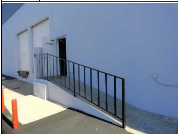
21. Exterior ramp and stairs on west elevation
