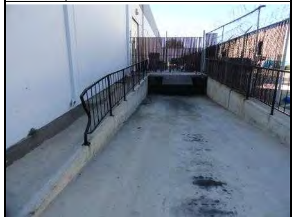
17. Exterior tailgate-high loading dock at the northeast corner of the building
