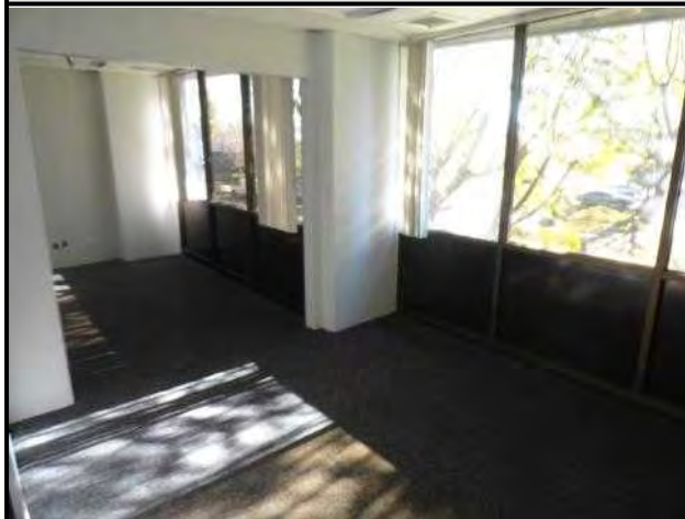
Second floor office area finishes
