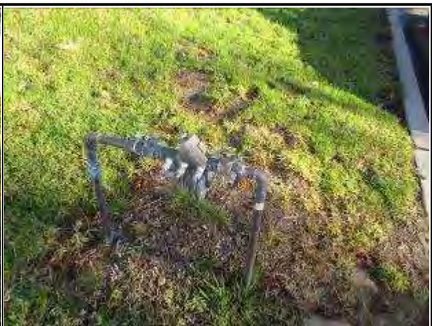
Figure 2.2.2 – Domestic water incoming service
