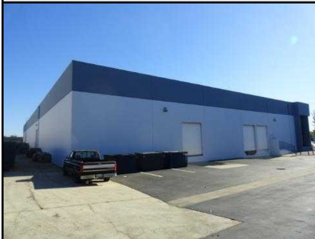
Tailgate high loading docks and concrete aprons along west building elevation
