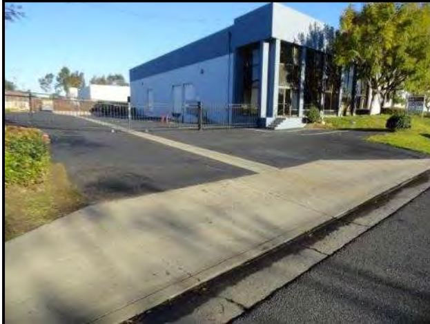
Storm water is directed off site to municipal systems
