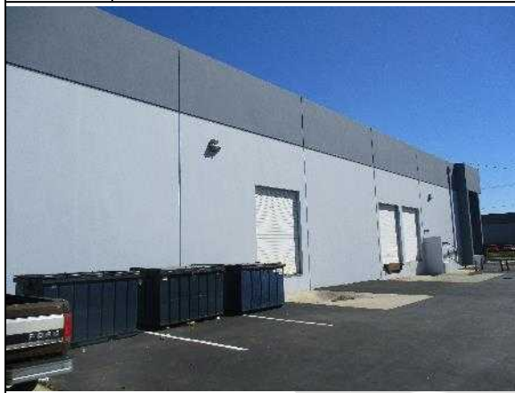
2. Representative façade with some loading dock doors.
