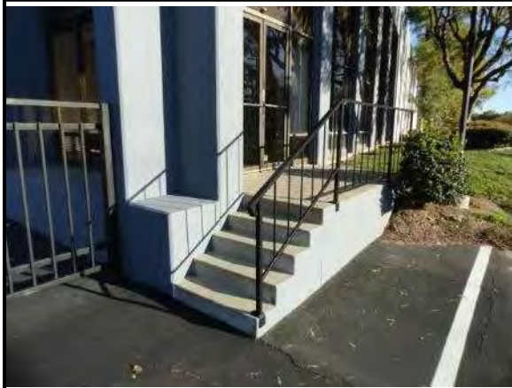
20. Exterior stairs at southwest entrance
