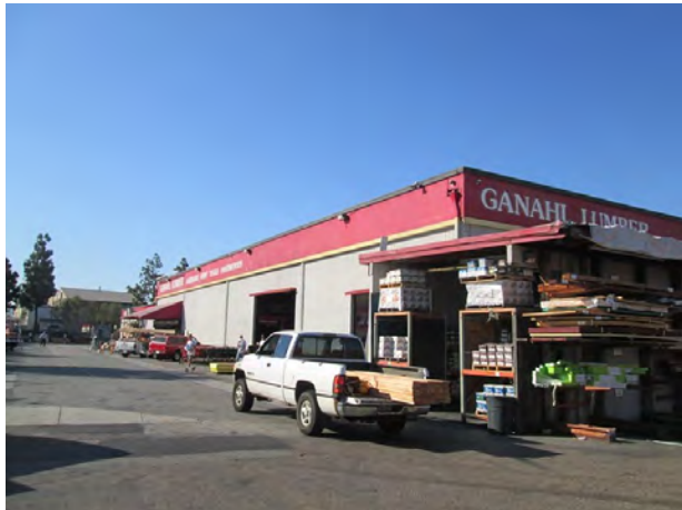
5. View of the northeastern portion of the subject property building.
