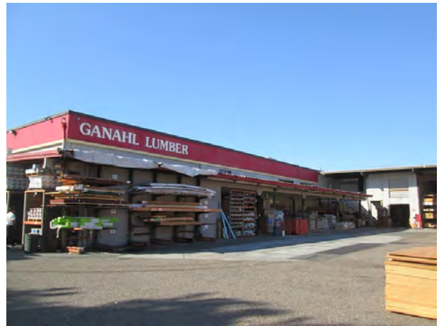
4. View of the northwestern portion of the subject property building.
