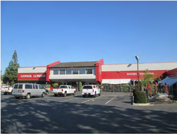
1. View of the southeastern portion of the subject property building.
