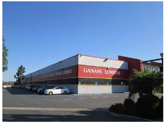
2. View of the southwestern portion of the subject property building.
