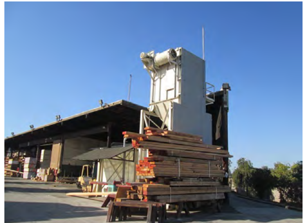
6. View of the northwestern portion of the subject property building.
