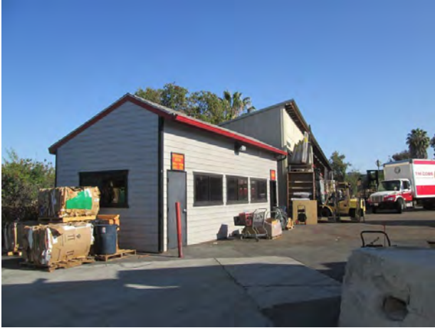
7. View of the operations office and storage shed located on the northwestern portion of the subject property.
