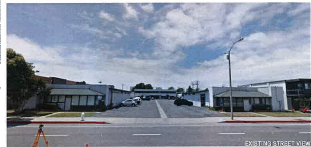
EXISTING STREET VIEW
