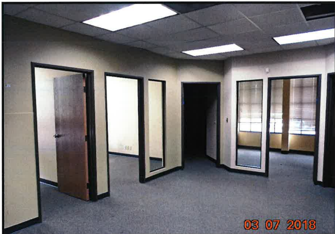
Existing Offices (to be demolished).
