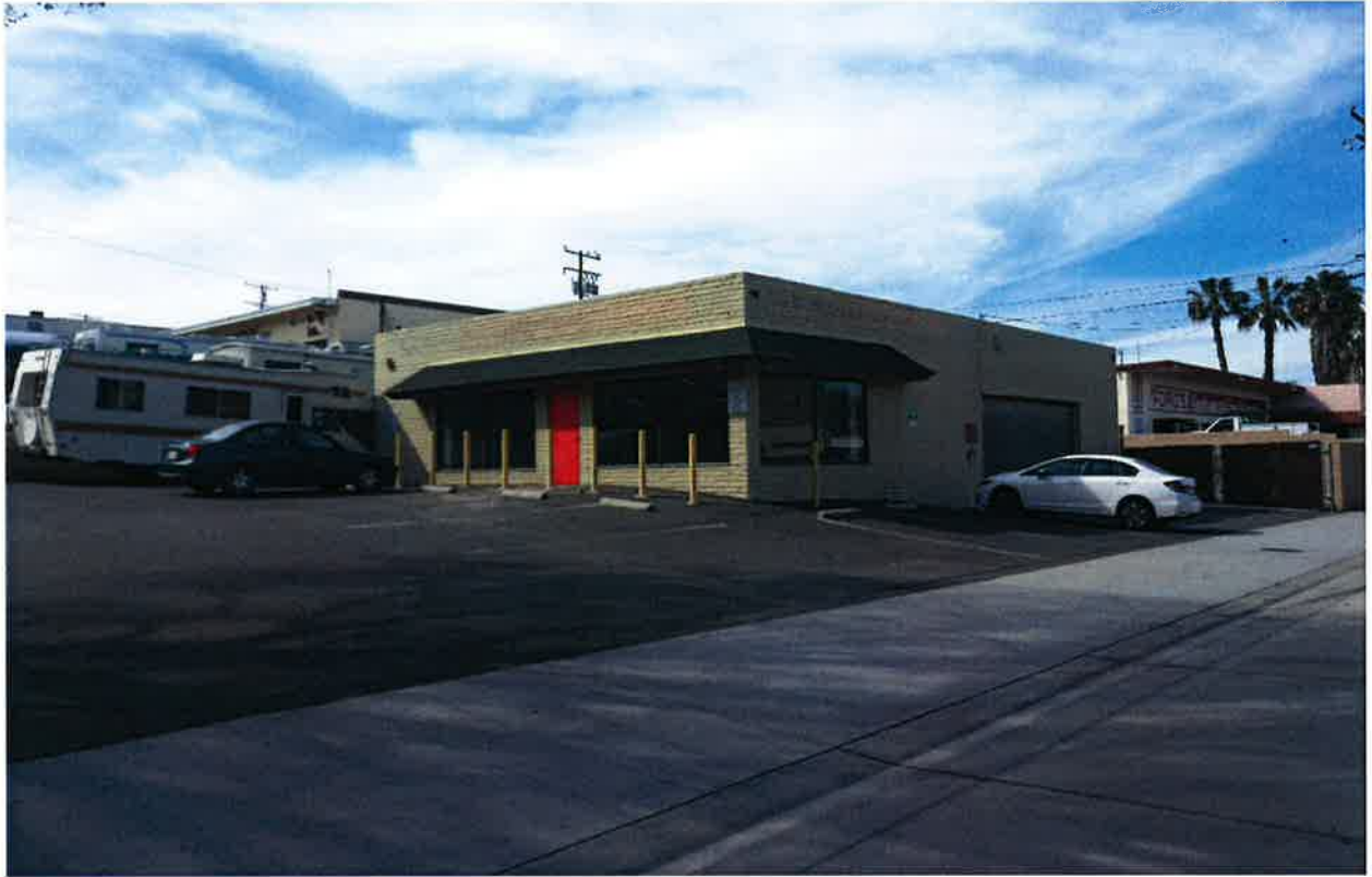
Northwest view of the subject property (704 W 16 th Street)
