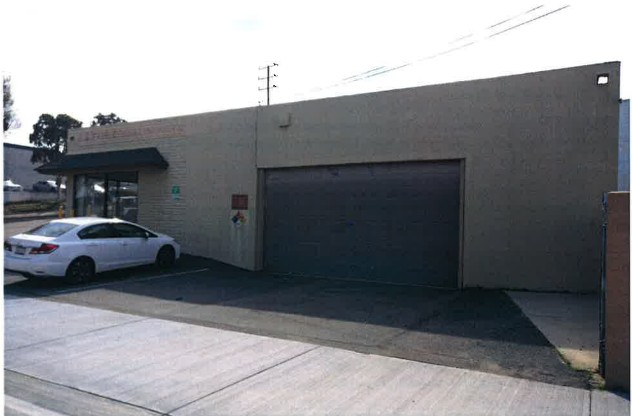
Side elevation of the subject property looking west
