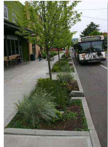
Green Infrastructure - Harvesting Rainwater(Brad Landcaster)
