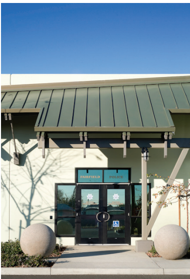
view at building entry
