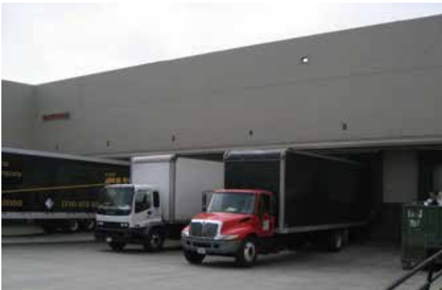
View of the elevated dock area at the Robinson Pharma space.
