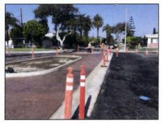
removal of existing asphalt pavement, curb and gutter, curb ramps, local depressions, sidewalk, excavation of unclassified material, grading and traffic control.
