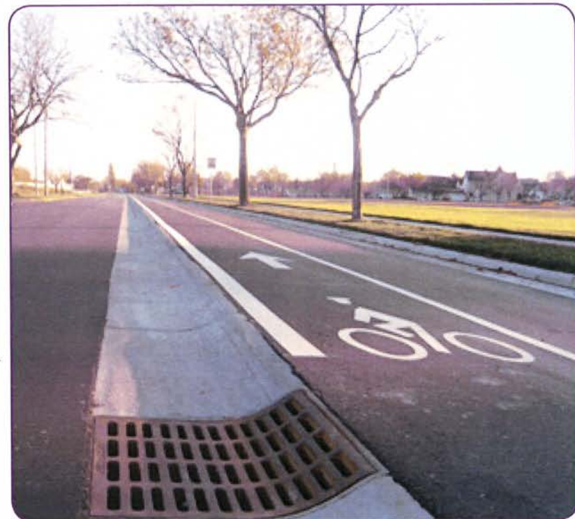
Figure 3-11 Class II Raised Bicycle Lanes
