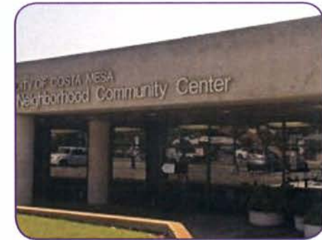
Figure 4-13 Costa Mesa Neighborhood Community Center
