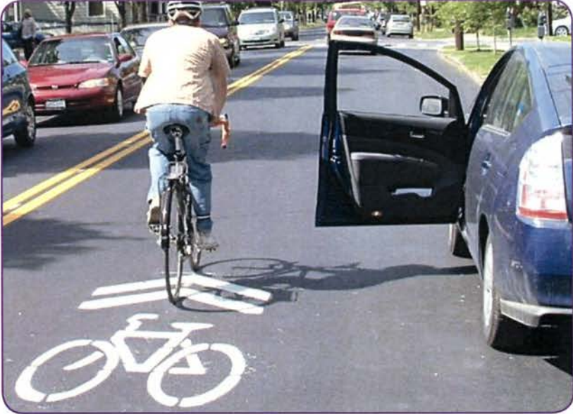
Figure 3-7 Lanes with Sharrow Marking
