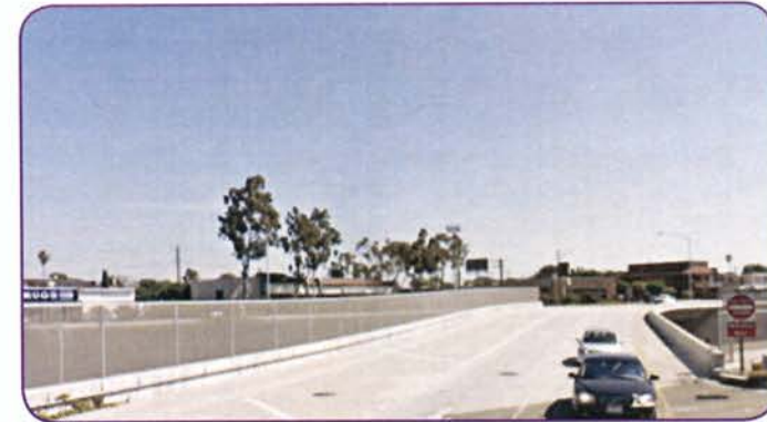
Figure 4-6 Looking south along the Fairview Road bridge over SR-55, wide striped shoulder visible
