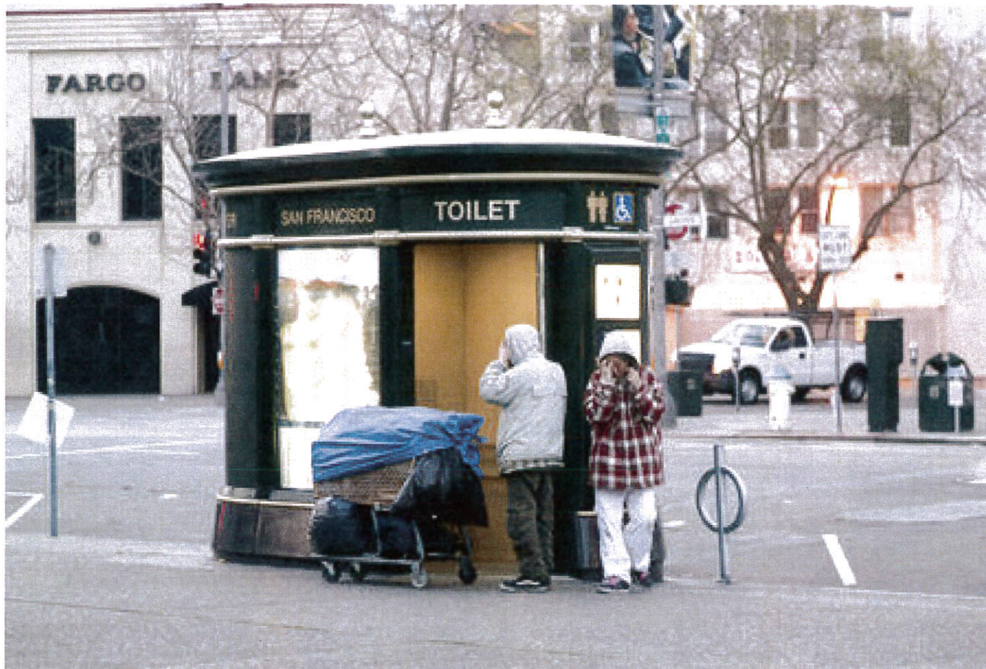
The public restroom near City Hall gets plenty of use. During business hours the units are havens of drugs and prostitution, and often filthy. Photo by Jason Winshell/SF Public Press.
