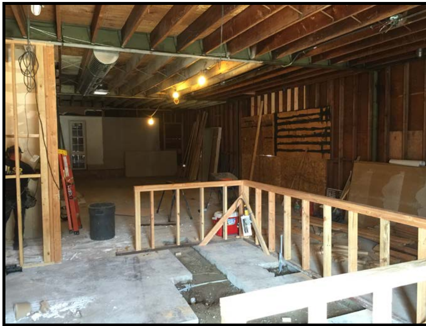
8/25/16 Photo of Red Room Under Construction (Future Bar Area in Foreground)
