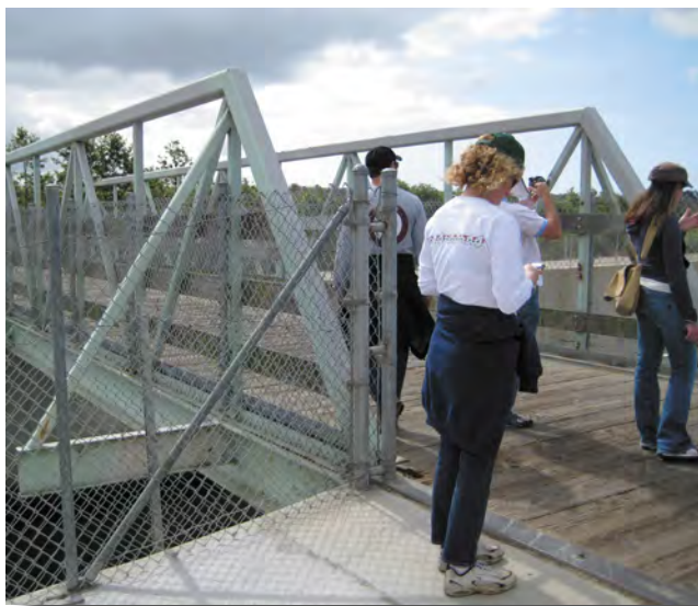
Figure 35: Greenville Banning Channel Bridge
